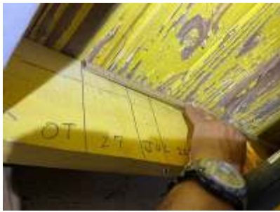
Two Nails per Board #1
