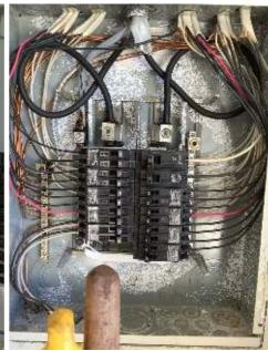
Branch Wiring Circuits, Breakers & Fuses: Branch Wire 15 and 20 AMP Copper
