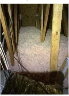
**Attic Insulation: Insulation Type**Blown, Fiberglass
