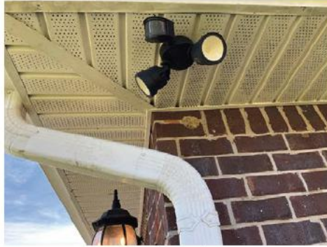
Soffit vents
