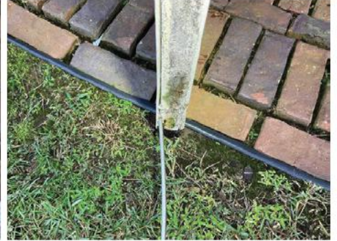
Shed door left side (also in WDO report)
