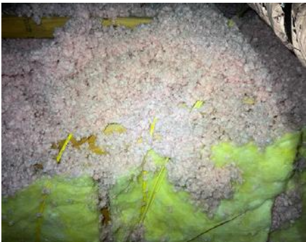
Attic Insulation: Insulation Type Batt, Fiberglass, Loose-fill
