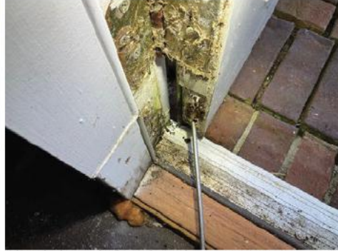
Shed door left side (also in WDO report)
