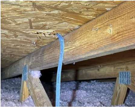
Attic Insulation: Insulation Type Batt, Fiberglass, Loose-fill
