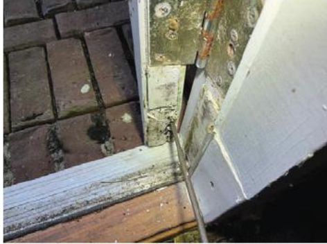
Shed door right side (also in WDO report)
