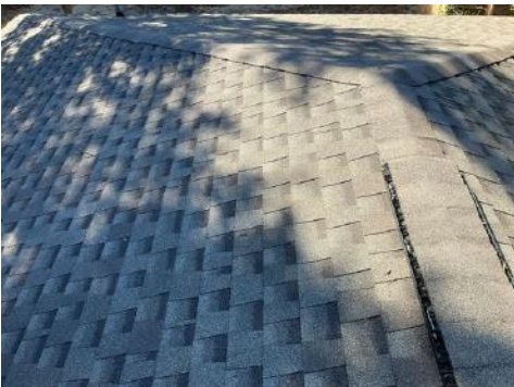
Photos of Each Slope
